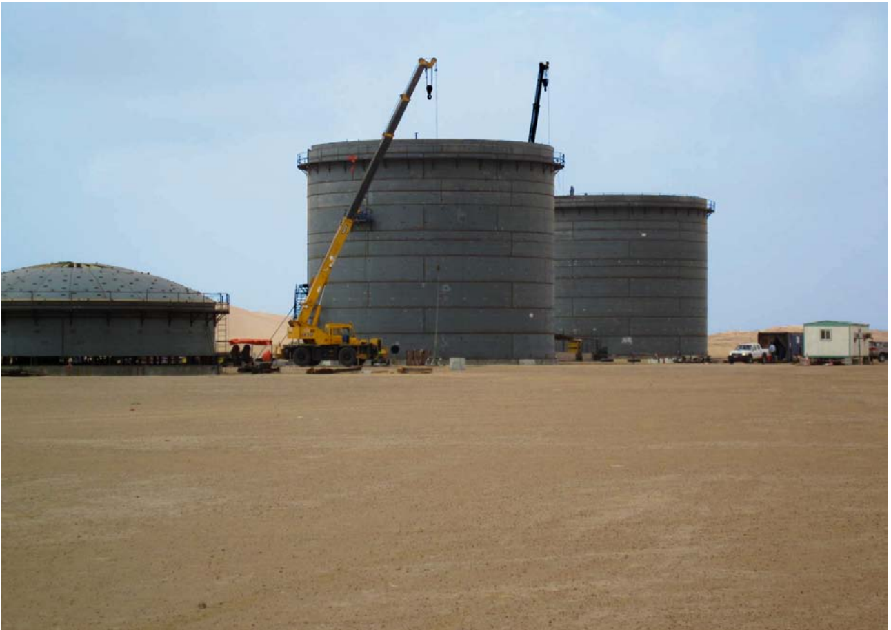
Saiwan site construction
